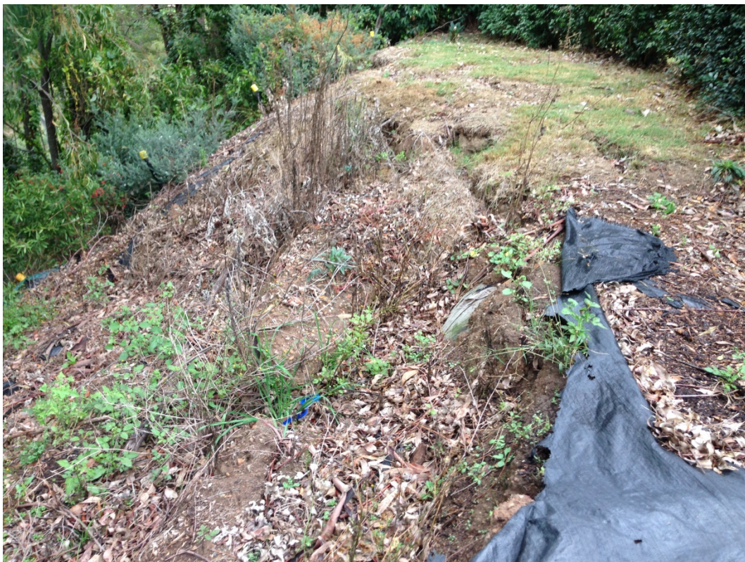
Figure 12 Tension cracking crest of slope 17 Staley Court
