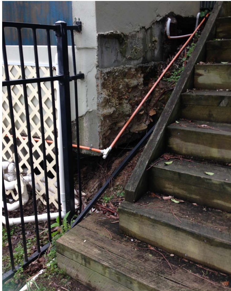
Figure 13 Loss of soil at base of pool foundation 19 Staley Court
